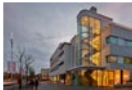
2 Bouwinvest MOVE & The Garage Rijnboutt, BiermanHenket, QuA Associates, Bronsvort Blaak Architecten (i.o.v. Pon)
